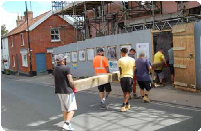
Eight-man team carry massive oak beam.
